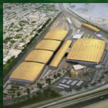
Rashidiya Main Depot, Dubai
